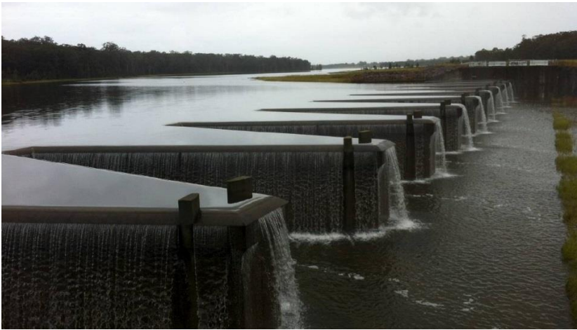
Figure 2-2 New Grahamstown Dam labyrinth spillway (source: Port Stephens Examiner, 2008)
