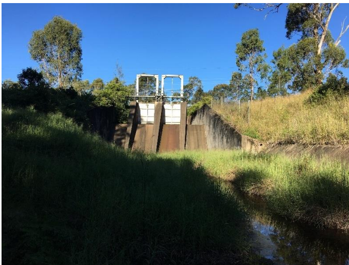
Figure 2-1 Original Grahamstown Dam spillway gates
